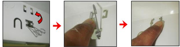
**Step 6:** Tie the holding spring (inner part of the lamp frame) as shown in the picture above.
