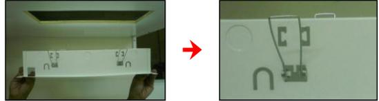
**Step 5:** Turn the spring (outer part of the lamp frame) to make it face upward when placing the lamp frame in the ceiling.
