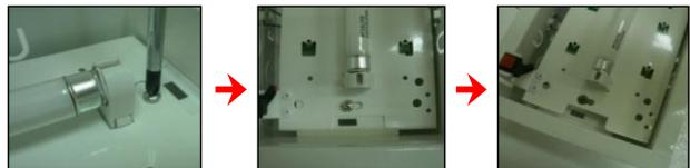
**Step 3:** Remove the control gear tray from the lamp frame after loosen the screw from its holder.
