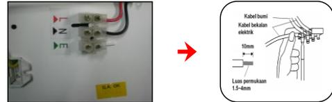
**Step 7:** Insert the electric supply cable to the provided connector.
