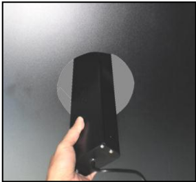
Step 4 : Connect the (male) connector from the transformer box to (female) connector from the lamp frame.
