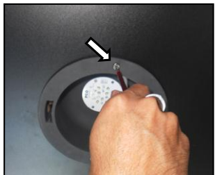
Step 5 : Insert the lamp frame into the ceiling hole and tighten both the screws according to the clockwise. Make sure the lamp cover is taken off before this step.
