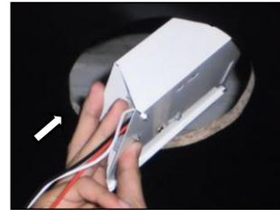
**Step 3 :** Place the transformer box into the ceiling after connect all the wires as in the above diagram.
