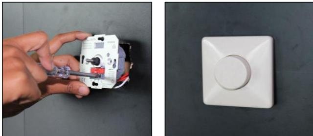
**Step 2 :** Connect the wires from the transformer box to the dimmable switch.
