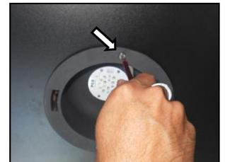
**Step 5 :** Insert the lamp frame into the ceiling hole and tighten both the screws according to the clockwise. Make sure the lamp cover is taken off before this step.
