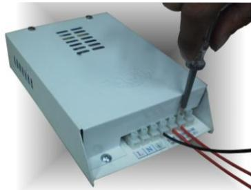
**Step 1 :** Connect the supply wires to the terminal block at the transformer box.
