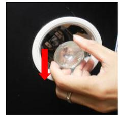
**Step 1:** Remove the cover by rotating it in the anti-clockwise direction.
