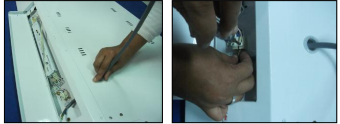
Step 4: Insert the electric supply cable into the lamp frame and connect it to the provided connector.
