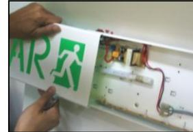
**Step 5:** Attach the diffuser with the lamp frame properly.
