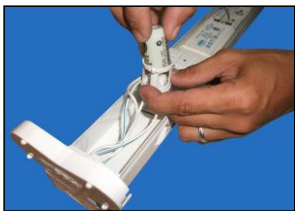
Step 3: Take Out starter from starter holder and attached at the prepared hole
