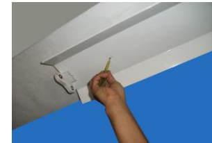
Step 7: Close the cover and place the reflector on top off the cover and screw with properly.
