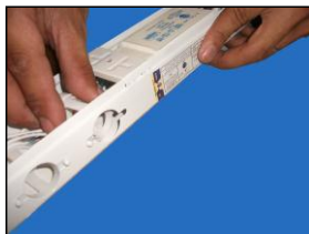
Step 3: Take Out starter from starter holder and attached at the prepared hole
