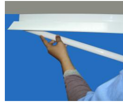
Step 8: Insert the tube properly and twist it 90°.
