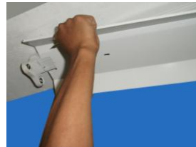
Step 7: Close the cover and place the reflector on top off the cover and screw with properly.
