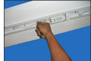
Step 5: Tie the fixture on ceiling after supply wire insert inside supply hole.
