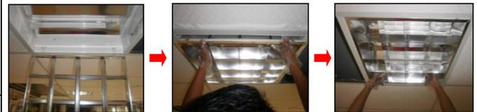
**Step 8:** After all the four clips are pressed, push the right side of the louver in to the lamp frame and followed by the left side. Then push the whole louver into the lamp frame.
