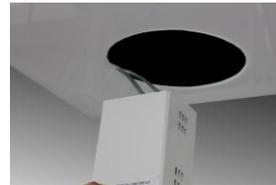
**Step 6:** Insert the transformer box into the ceiling and place it properly.
