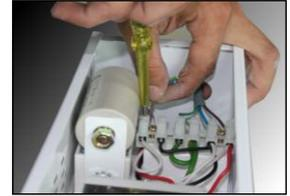
**Step 5:** Connect one more cable from the transformer box to connect to the lamp compartment then close back the cover.
