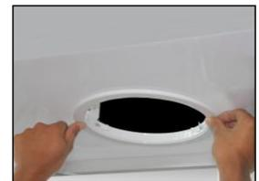
**Step 8:** Insert the fixture into the ceiling and lock it with nylon cap screws.
