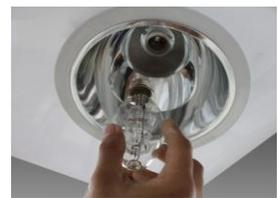
**Step 9:** Insert the reflector properly into the fixture then install the lamp by screw it until tight.
